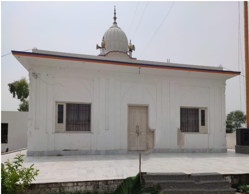
Illustration 5.9 A Structure of Gurudwara raise over the Samadhis of Gurmukh Das and Jawahar Singh Source: Author
