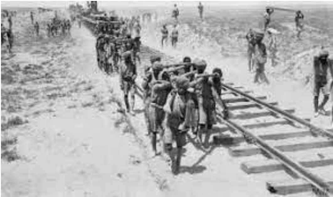
The Indian Labour Corps (ILC) laying railways tracks in the Middle East.
