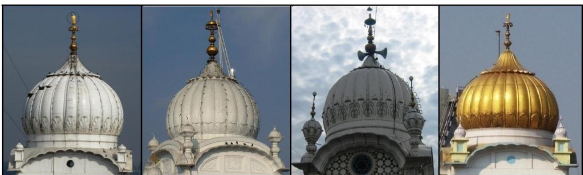
Figure: Domes of Gurdwara Bhatta Sahib, Katalgarh Sahib and Fatehgarh Sahib at Fatehgarh Sahib
